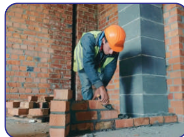
PLUMBER WORK MASSON WORK
